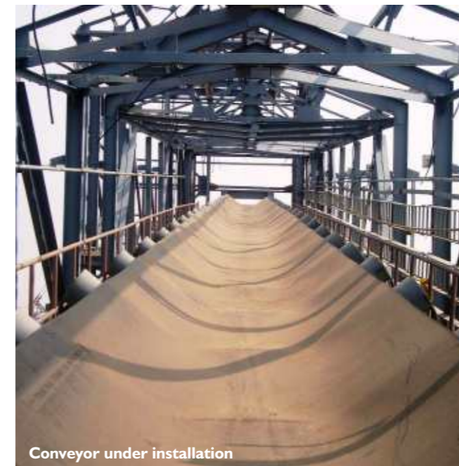
Deep bucket conveyor for hot clinker in cement plant in Veraval
